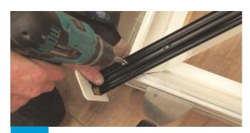
Fix each side of the hip glazing seat into the ringbeam flaps.
