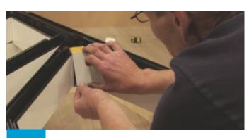
Where there is no bell rafter, glue internal ridge end caps onto each end of the ridge.
