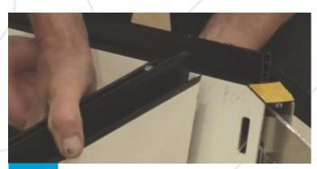
Locate into position with the top rafter bracket and tighten the screw.
