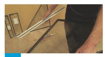
Glue packers into the bottom of the glazing end closer. Slide glazing end closer over the bottom of the glazing.
