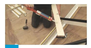
Silicone the foam board securely into place.
