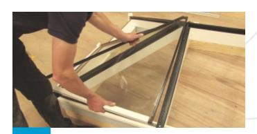
Fit all units of glass keeping glazing end closer between rafters.
