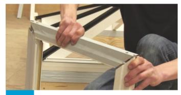
Remove one side of the roof vent sash.
