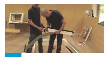
Engage the rafter bracket into the slot provided on the ridge.
