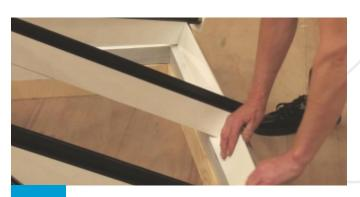
Before fixing the central and jack rafters at the bottom, temporarily fit foam boards against flap to correctly space rafter positions.
