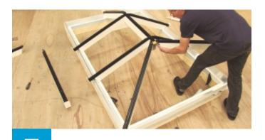
Fix the next hip and secure screw at top.
