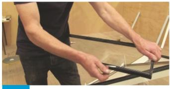
Remember to clear both sides and always use the correct sealant. Remember to remove tape from both sides.
