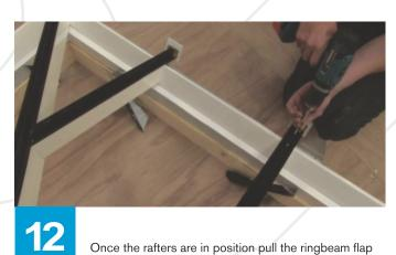
Once the rafters are in position pull the ringbeam flap up tight to the rafter and fix centrally with a screw.
