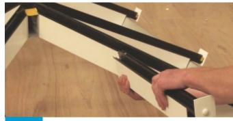
Jack rafters are located into a slot with a bracket and top screw.
