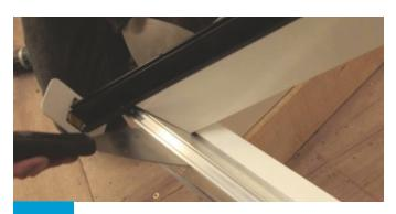
Rotate the ringbeam flaps keeping them tight against the hip rafter cut.
