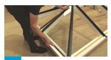
Lift glass into place behind the rafter end stops and press down glazing.
