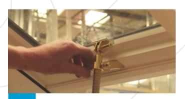
Locate the spindle and tighten bolts to secure.
