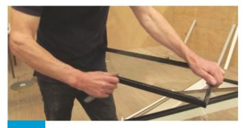
When fitting roof vents always remove foiled or plastic tape from surface of units before sealing.
