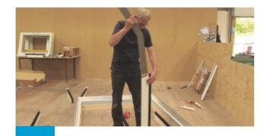
On a hidden tie bar push the steel bracket into the side of the central rafters.
