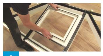
Locate the roof vent outer frame between the rafters.
