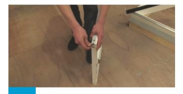
Loosen grub screw on sash corners with an allen key prior to glazing roof vent.
