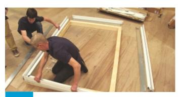
Lift the ringbeam onto the top of the kerbs. Make sure the ringbeam is sealed to the kerb base.
